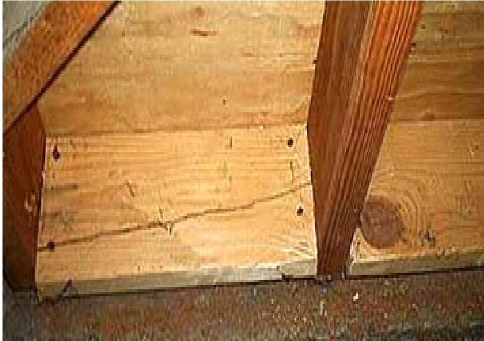
The photo above shows a block behind a shear wall that split with only four nails installed.
